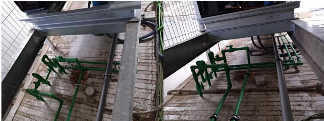
Mounting pipes with bypass in covered shed
